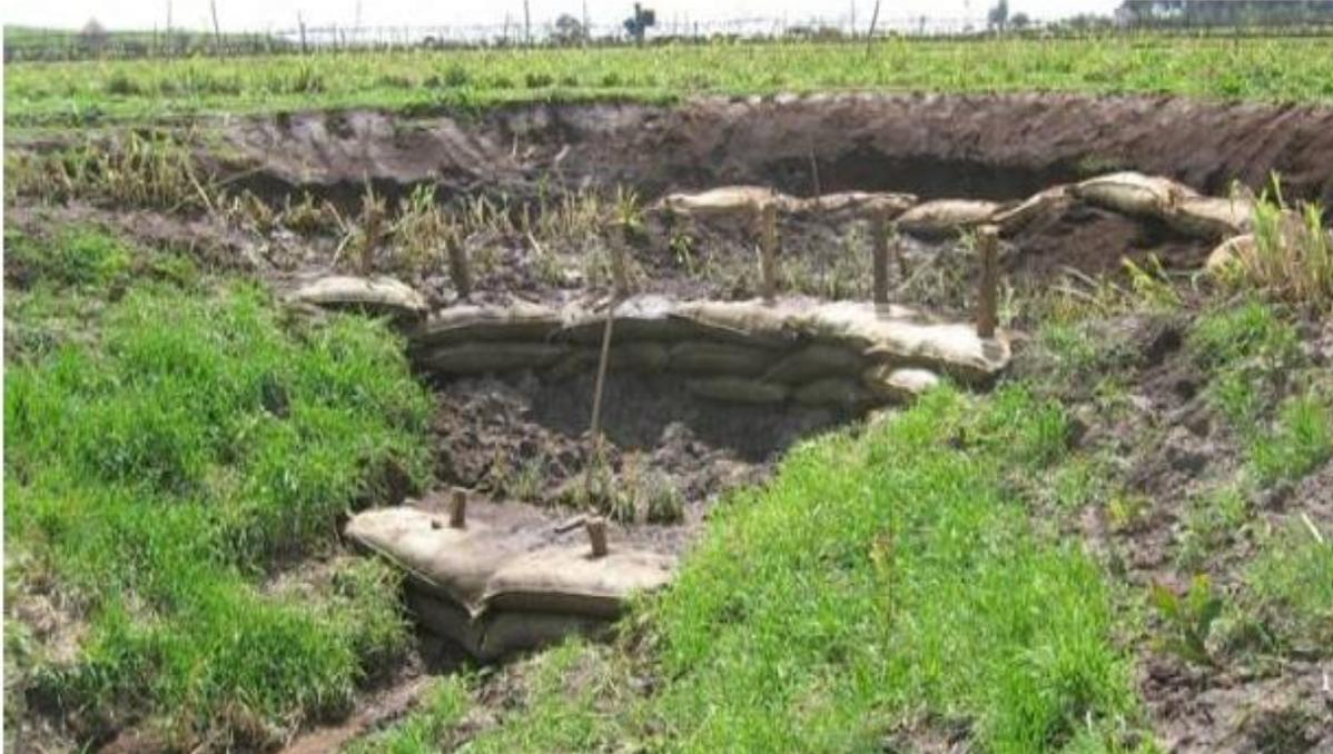
Figure 84. Sand/soil bag checkdams for gully stabilization in Amhara Region
