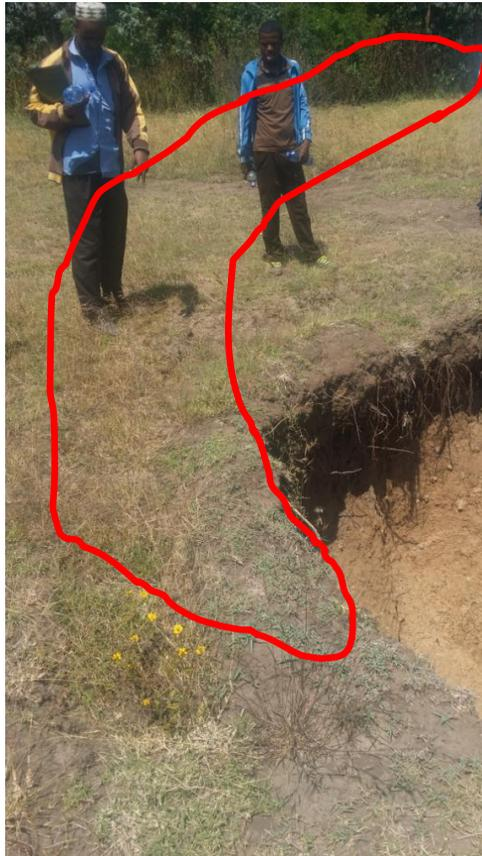
Figure 73. Canal dug above the gully head to stop its progressive development in Weteta kebele of Sankura Woreda
