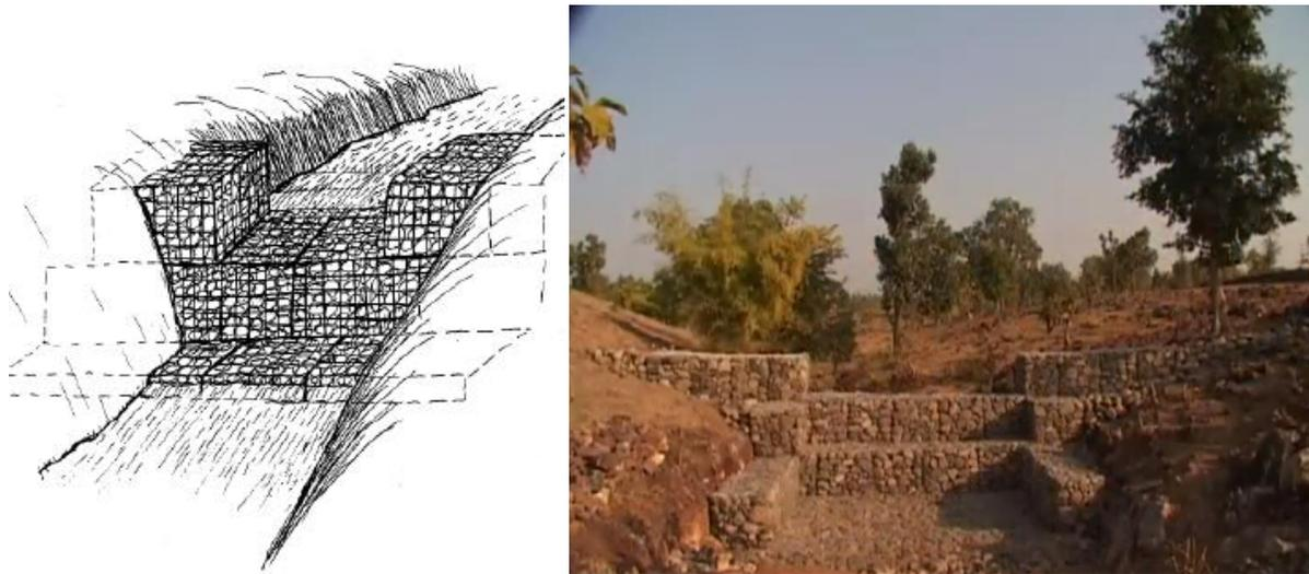
Figure 80. Gabion box checkdams (Source: Manual of Reforestation and Erosion Control, Agpaoa *et al.*, 1975)
