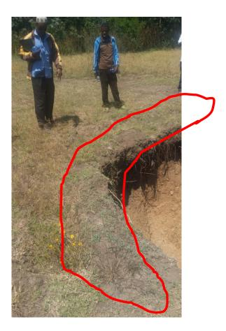
Figure 95. Canal dug above the gully head to stop its progressive development in Weteta kebele of Sankura Woreda
