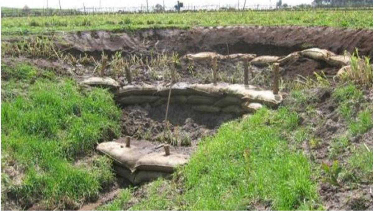
Figure 106. Sand/soil bag checkdams for gully stabilization in Amhara Region
