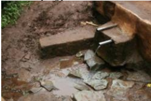
Photo 5.2: Spring protection in Aleta Wendo
