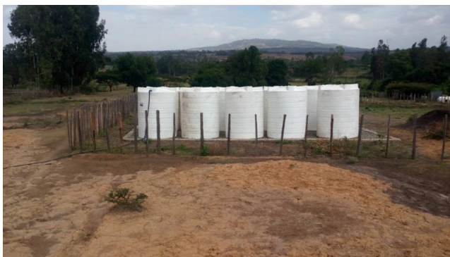
BO 104 – Accumulation System 250 m 3
