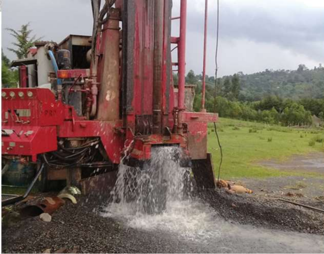
The drilling of borehole at Hamesho Kebele in Sidama Zone, SNNPR.
