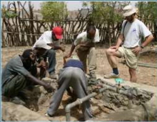
Technicians of GSE measuring the depth of a well at Humera, while supervised by Mr. Martin Hrubec from the Czech Ministry of Environment.
